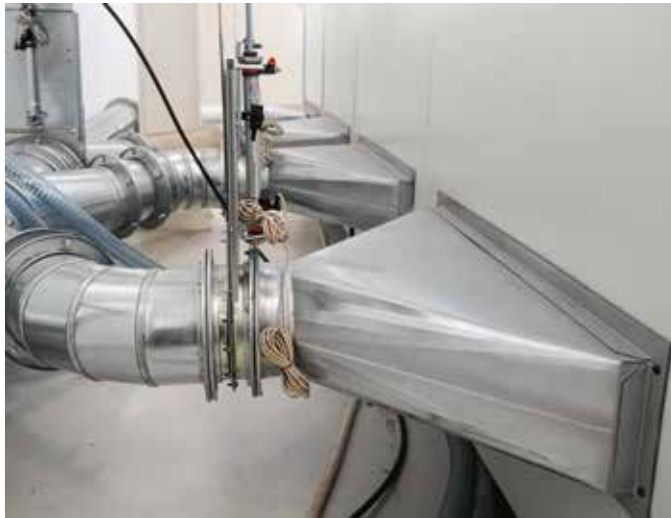
Dust extraction system for effective air change and dust abatement within the work area
